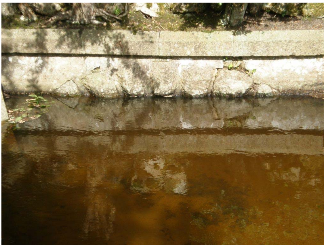
Plate 92 – Crown of mill race arch, now submerged but still taking water
