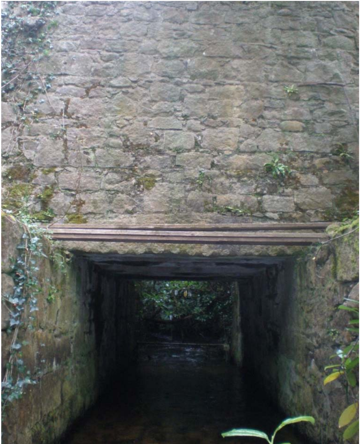
Plate 21 – Western elevation of Mill Race Bridge, note plug and feather marks on lintel
