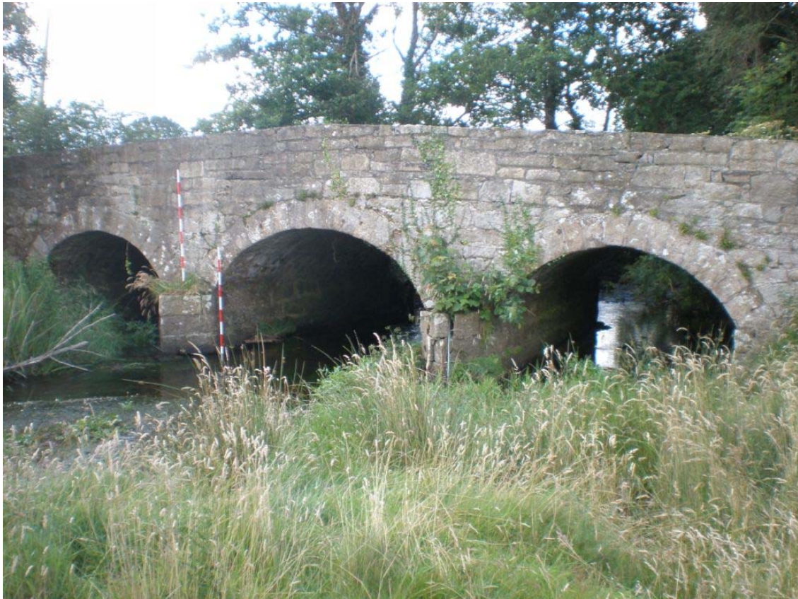
Plate 73 – Three true arched bridge at Dunroe Bridge, with later parapet also visible
