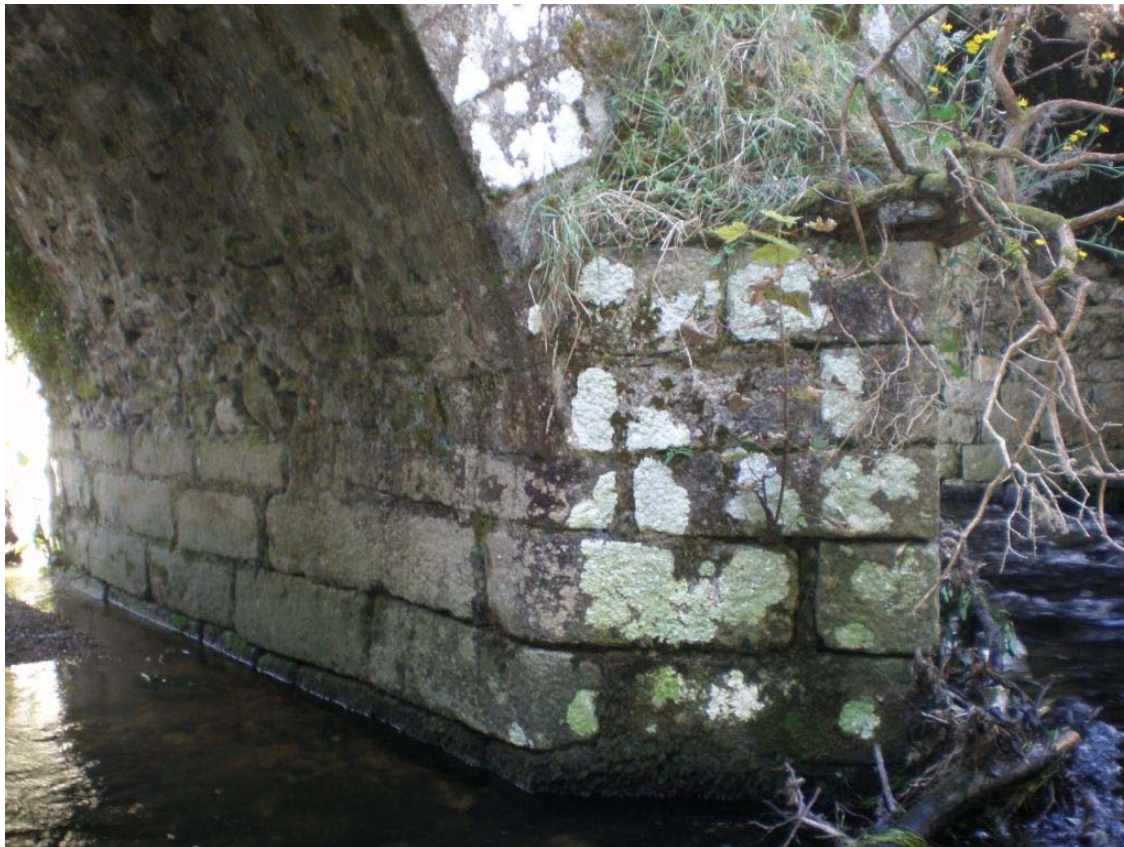
Plate 8 – Granite pier and cutwater with shale barrel in background
