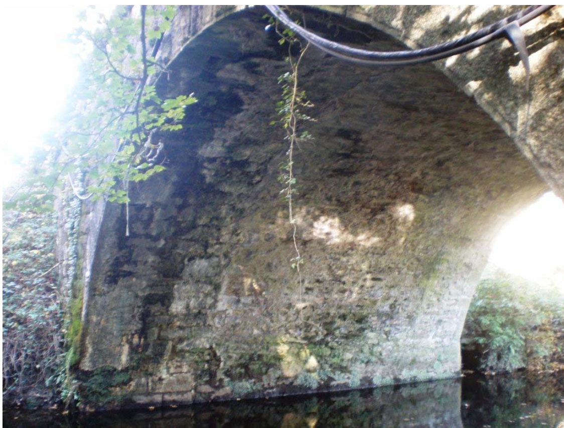
Plate 17 – Barrel of Ballycoppigan Bridge, note difference between east and west side
