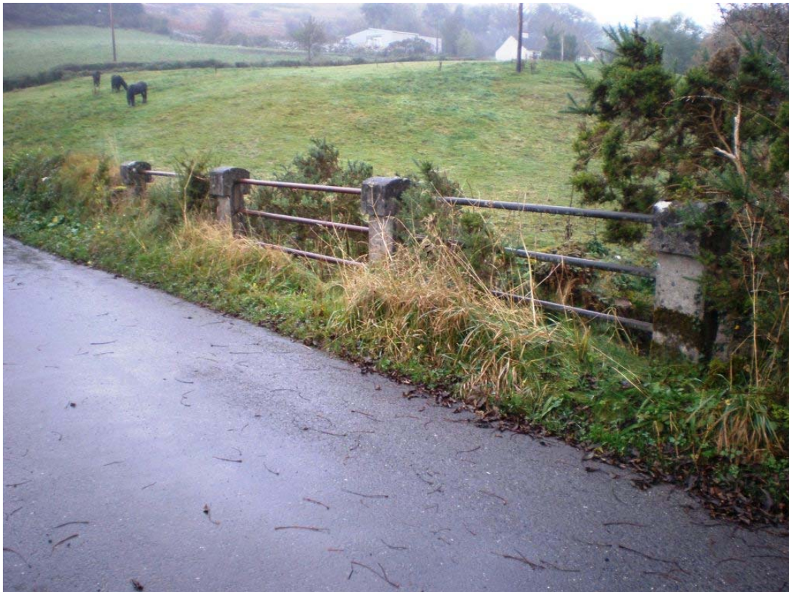
Plate 49 – Tubular railing and concrete post parapet
