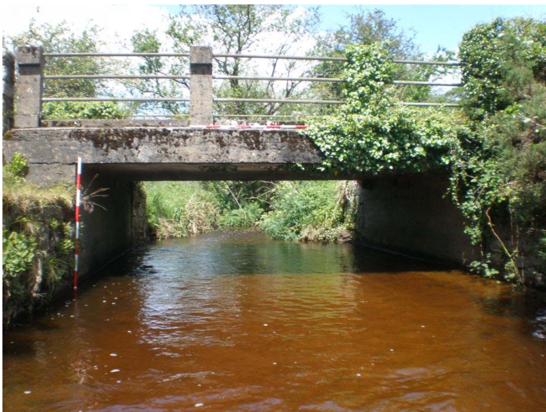
Plate 71 – Southern elevation of trabeated bridge at Knockullard
