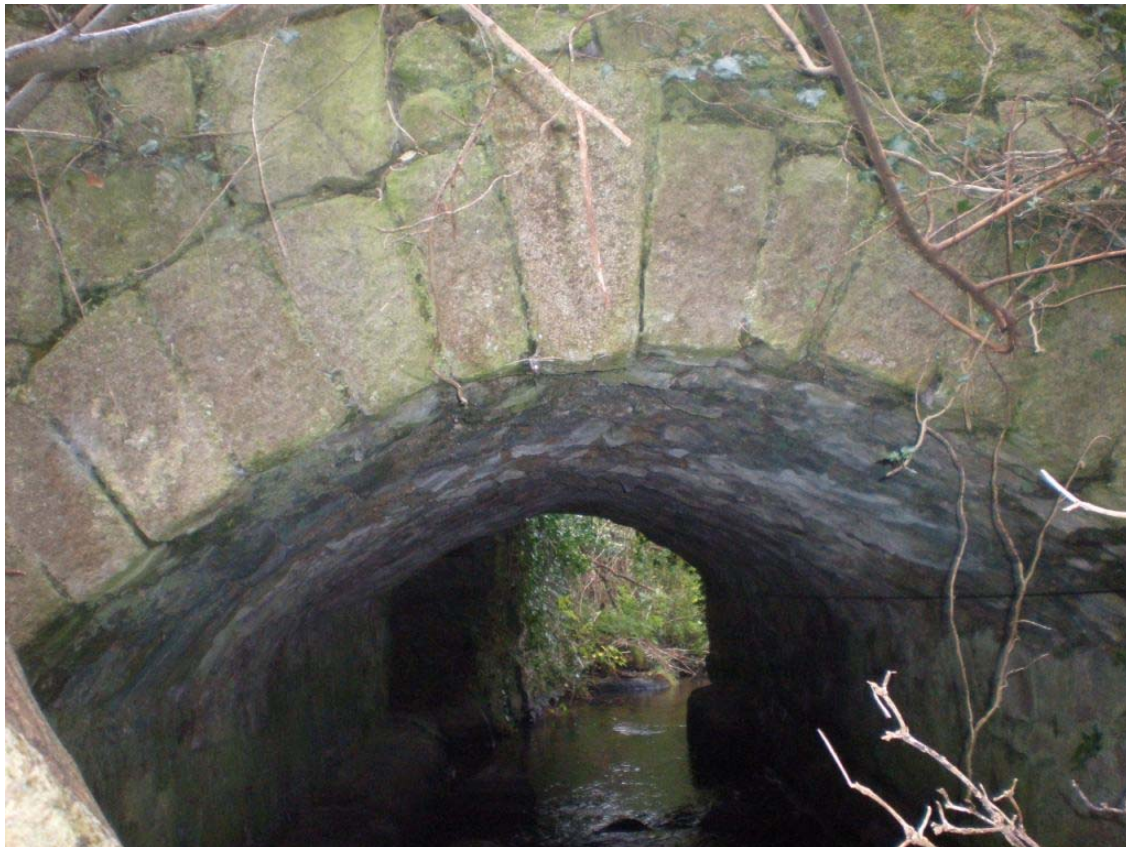
Plate 56 – Northern elevation of Coolnacuppogue bridge, with central keystone
