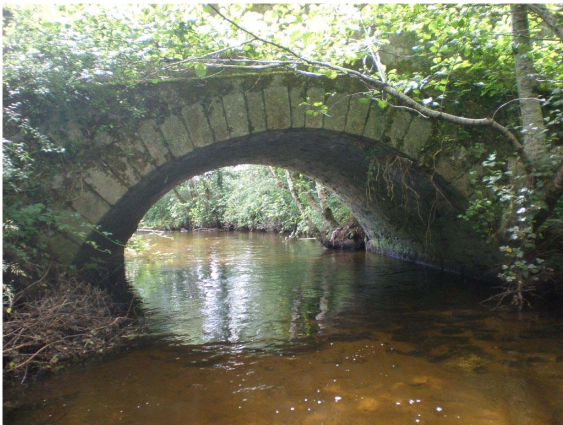
Plate 79 – Perfect true arch and barrel at Boley Bridge, with dressed voussoirs
