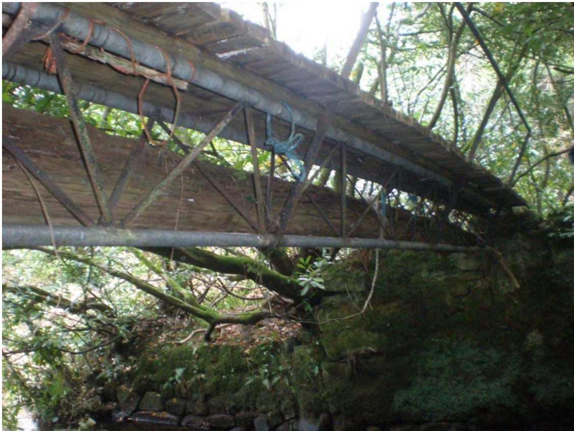
Plate 24 – Tubular steel framework for bridge
