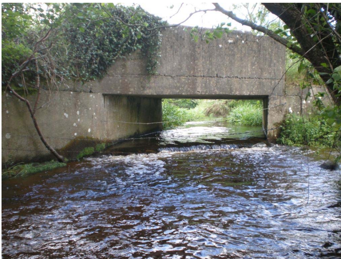
Plate 66 – Southern elevation, with concrete abutments and base evident
