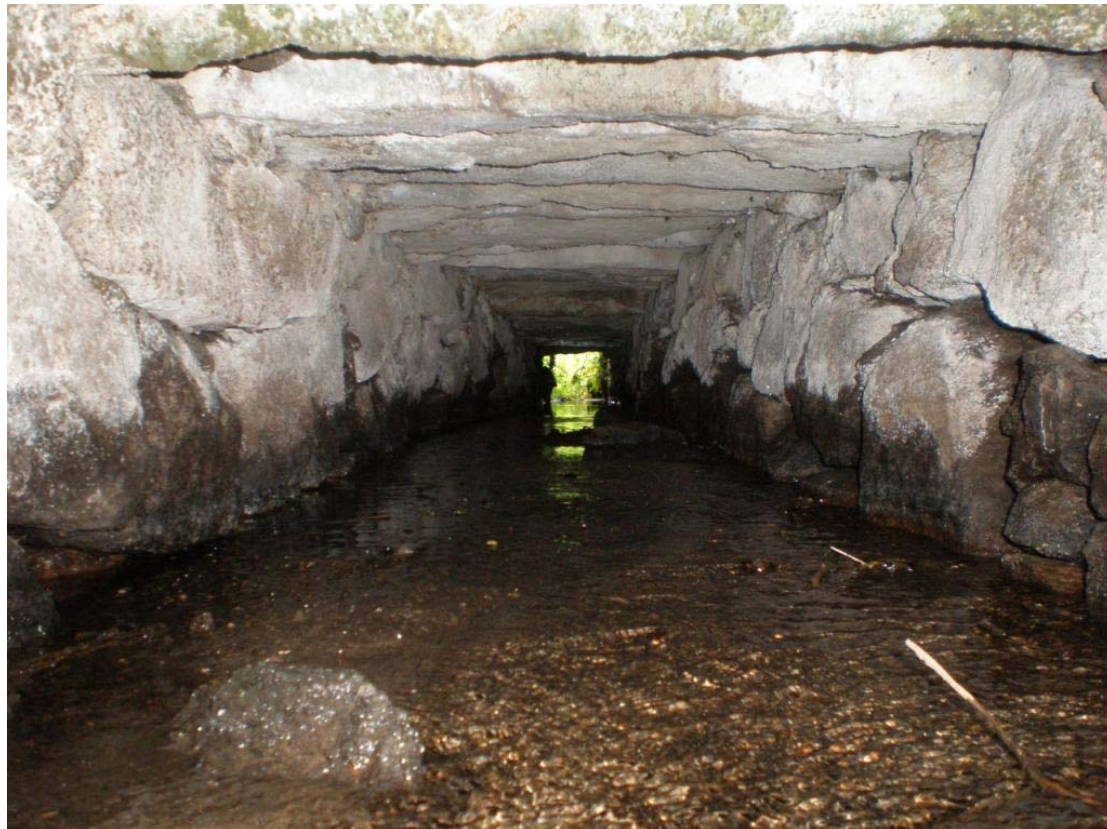
Plate 54 – Channel with granite abutments and lintels
