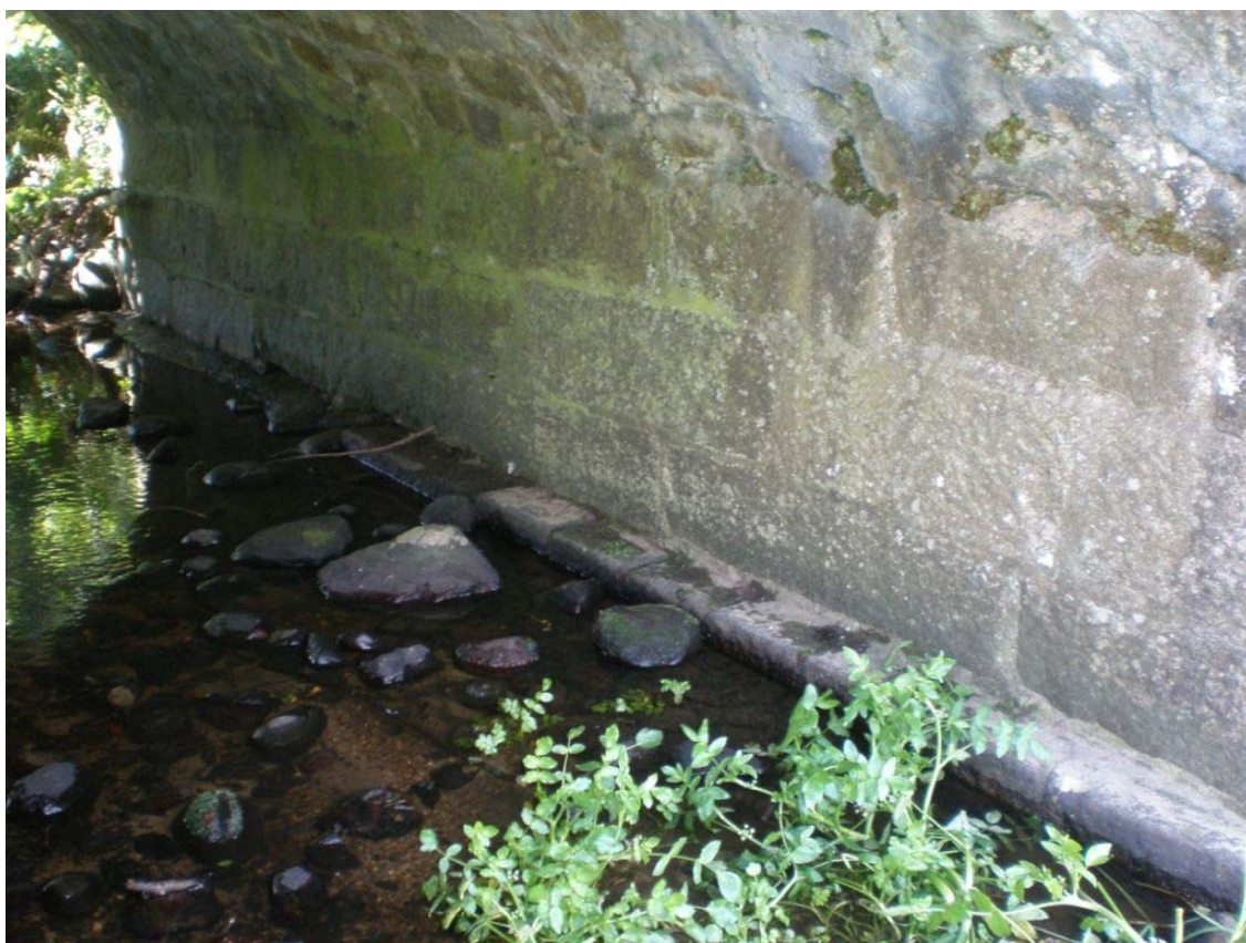
Plate 74 – Granite ashlar support on proud foundation course
