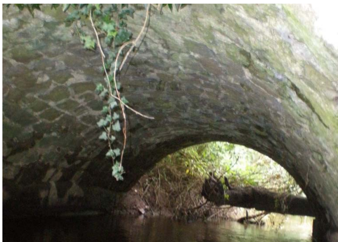
Plate 86 – Random rubble and dressed stone of the barrel
