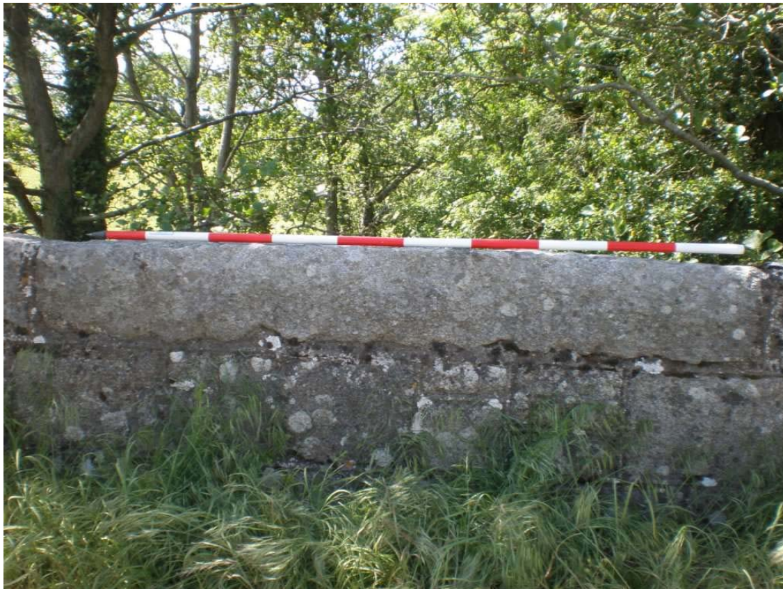
Plate 70 – Large coping stone of parapet, 2 metres long
