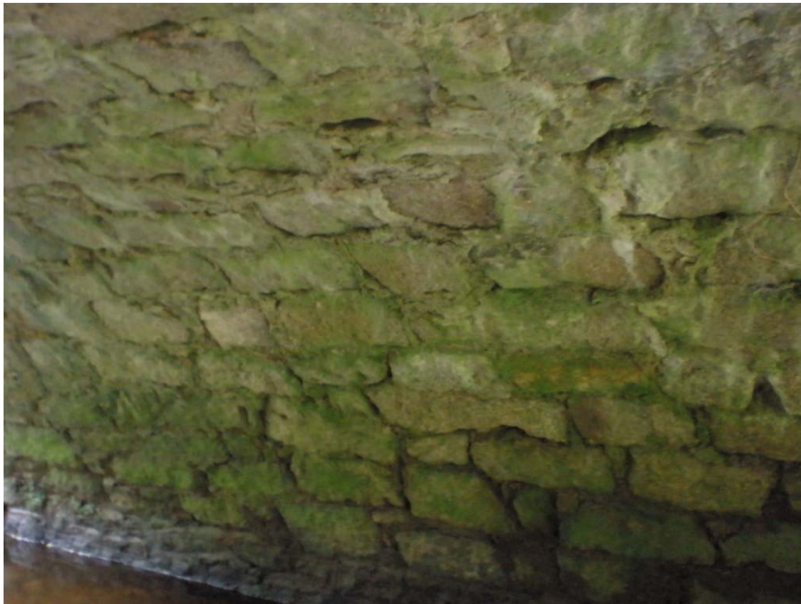
Plate 80 – Dressed granite within the barrel at Boley Bridge
