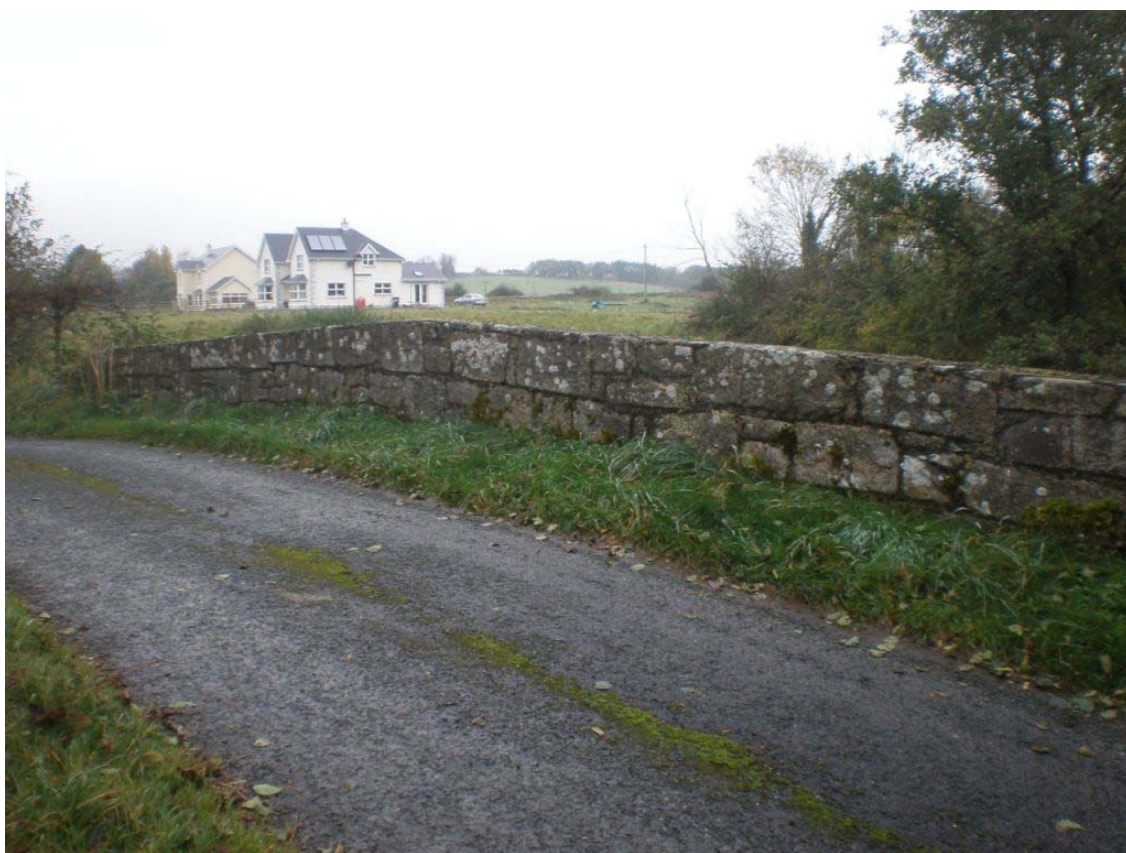
Plate 75 – Later parapet wall constructed in the 1950s
