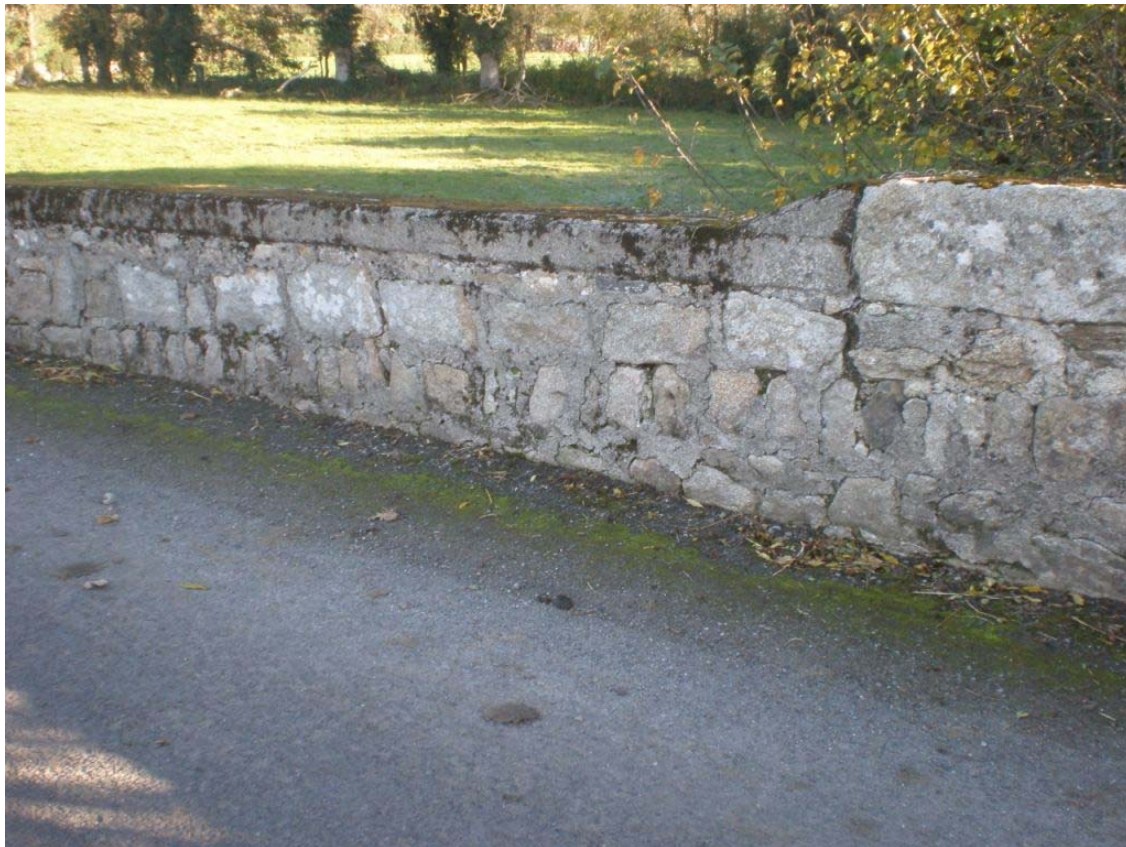
Plate 43 – Original bridge coping (sloping line) within parapet wall of later extension
