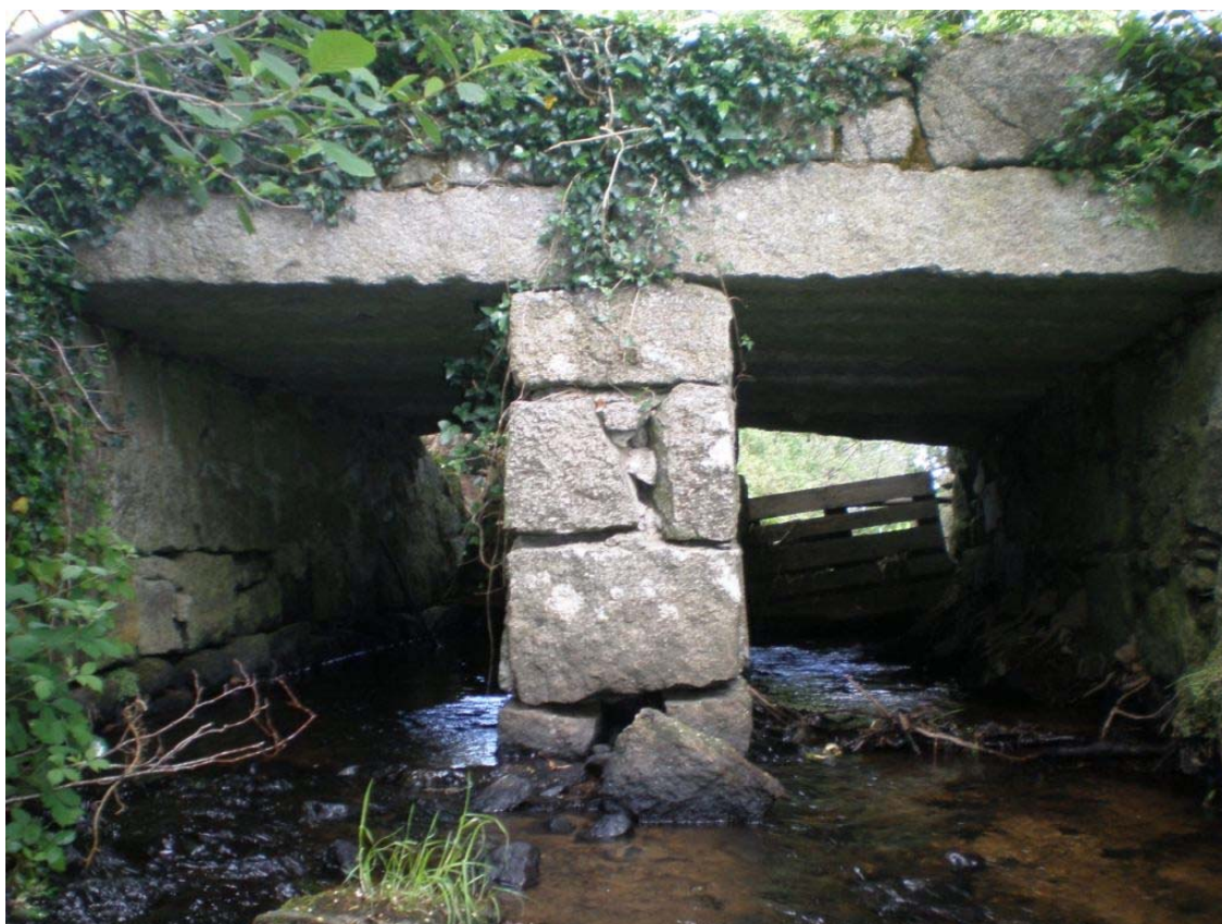
Plate 57 – Western elevation of bridge, note the plug and feather marks on the lintels
