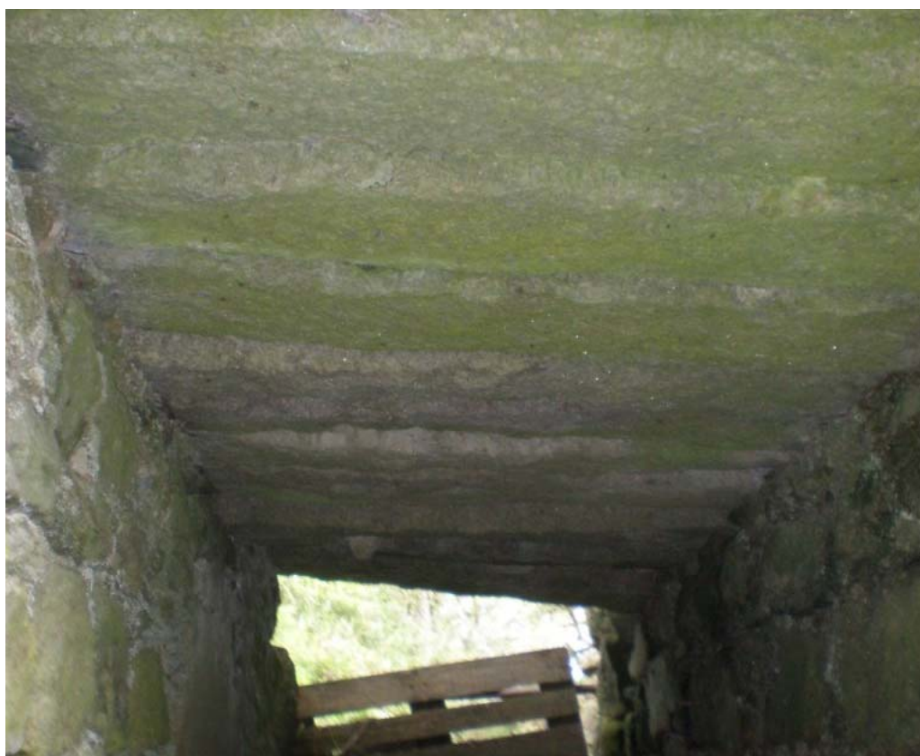
Plate 58 – Soffit of the arch, with individually dressed granite lintels
