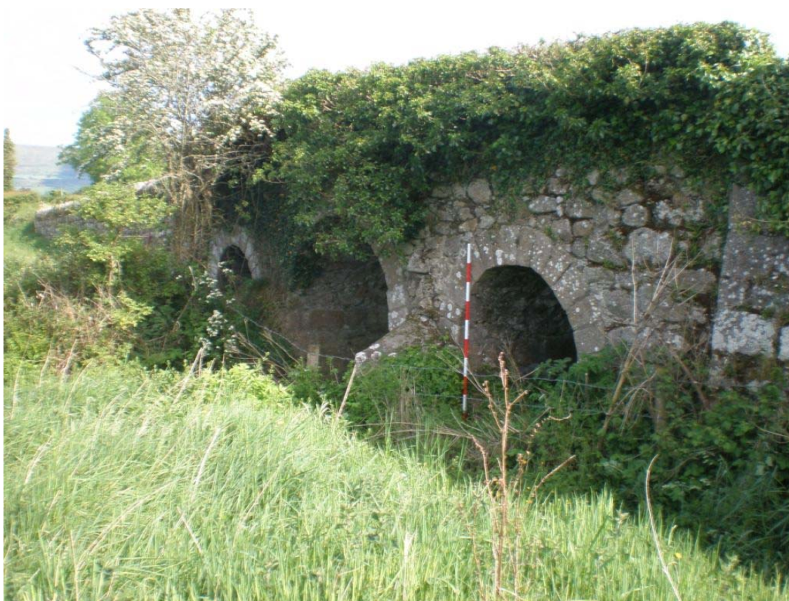
Plate 59 – Northern elevation of Aughabeg Bridge showing the three true arch spans
