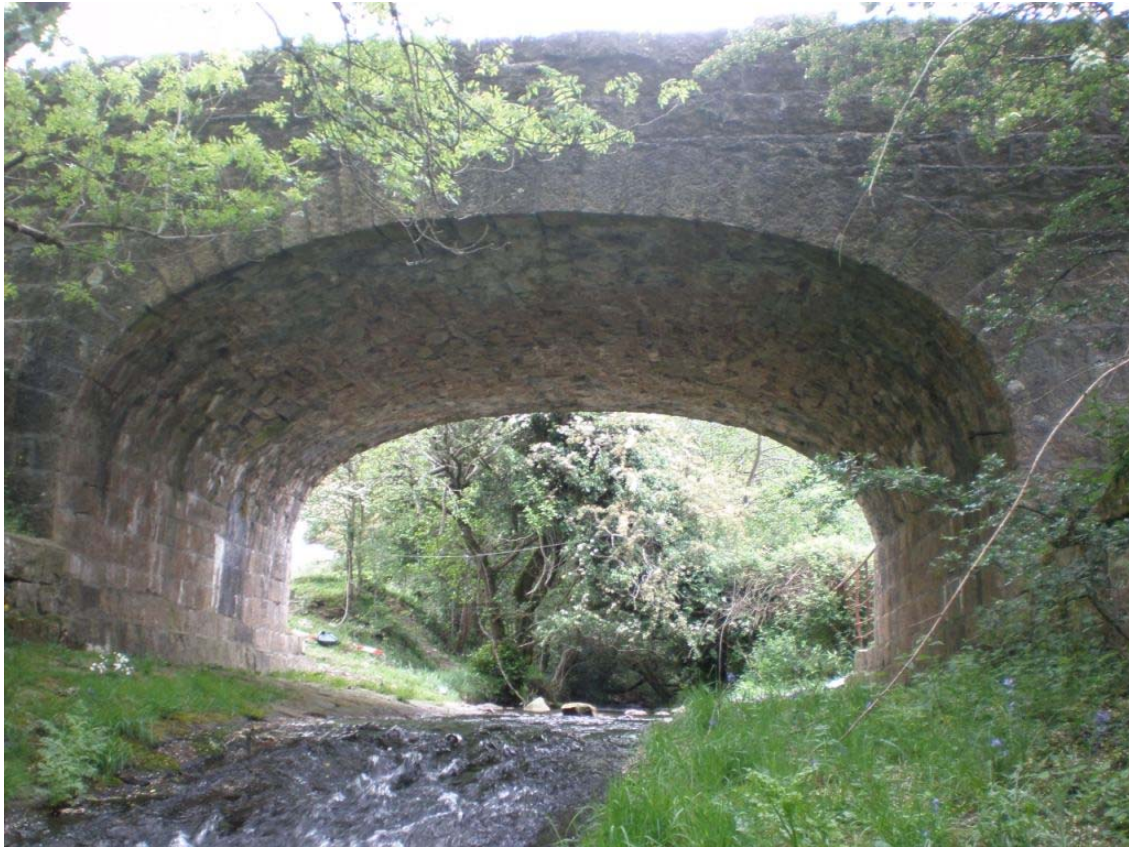
Plate 38 – South-western elevation of Kelly’s Bridge, note the high springing point
