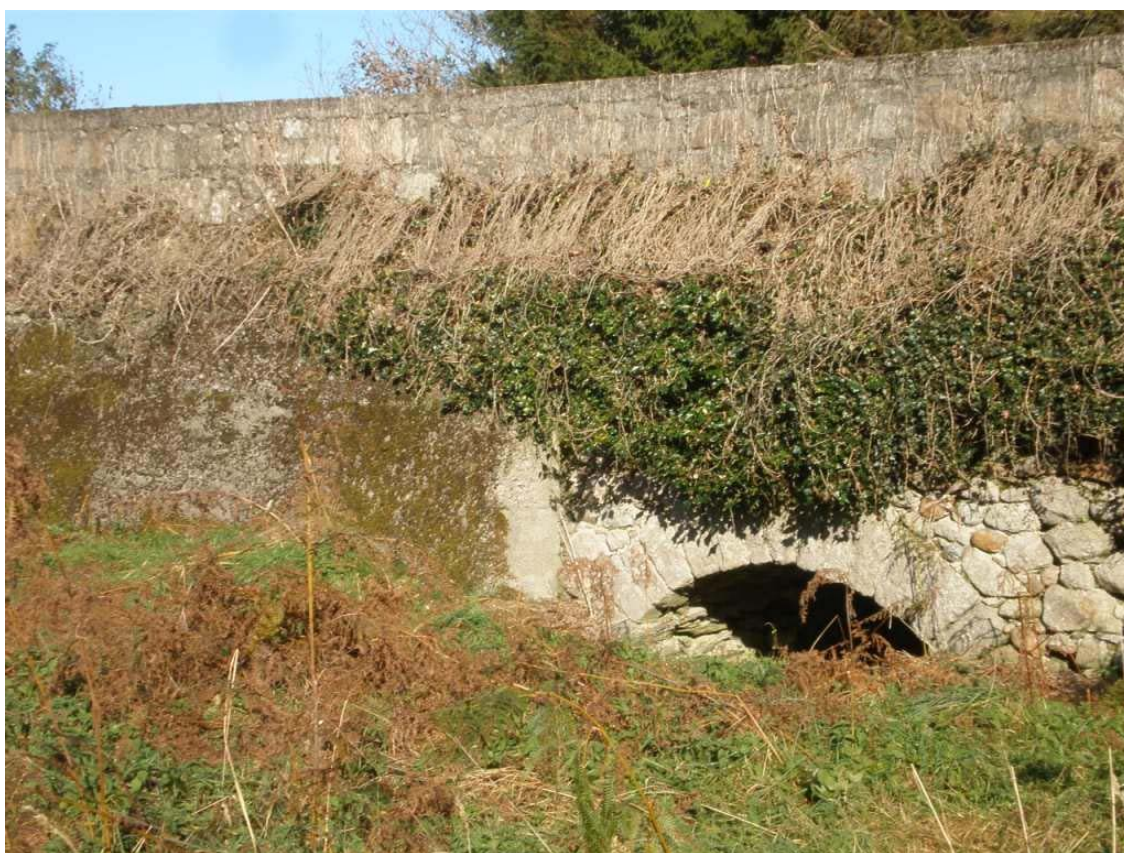
Plate 10 - Arch and later concrete abutment on south-eastern elevation
