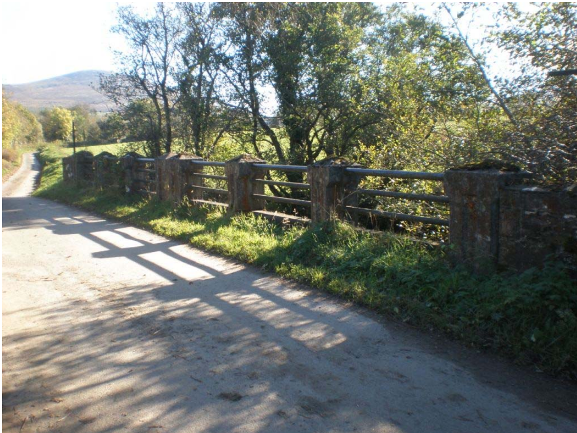
Plate 7 – Concrete post and tubular steel parapet
