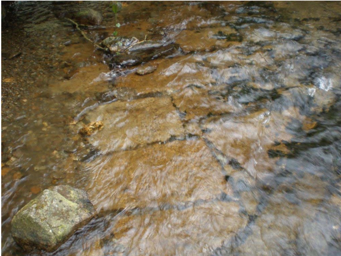
Plate 37 – Granite paved river bed
