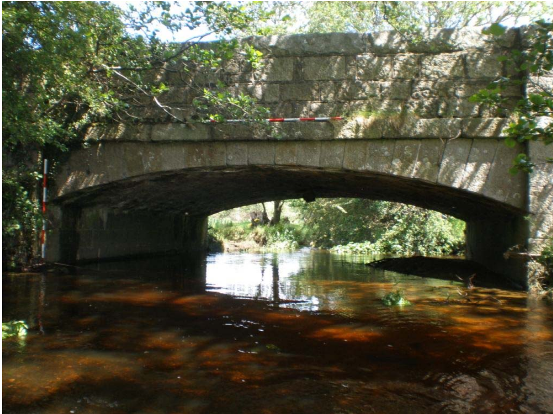
Plate 68 – Corries Bridge, with finely dressed voussoirs, string course, parapet and coping
