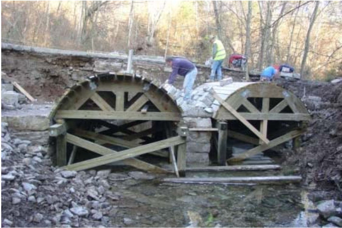
Plate 98 – Bridge construction using timber centring courtesy of http://www.drystone.org/
