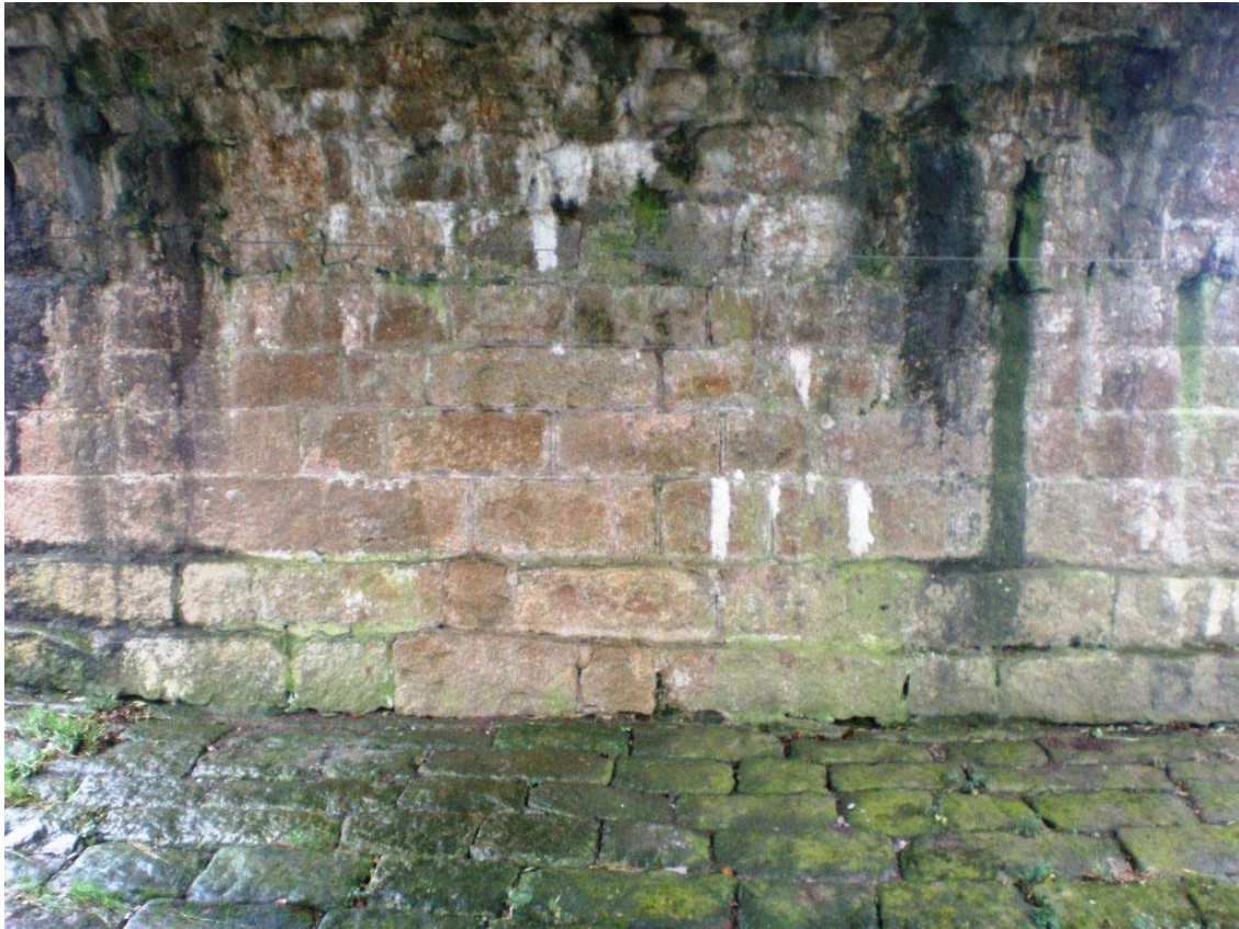
Plate 40 – Granite paving, foundation courses and abutment of Kelly's Bridge
