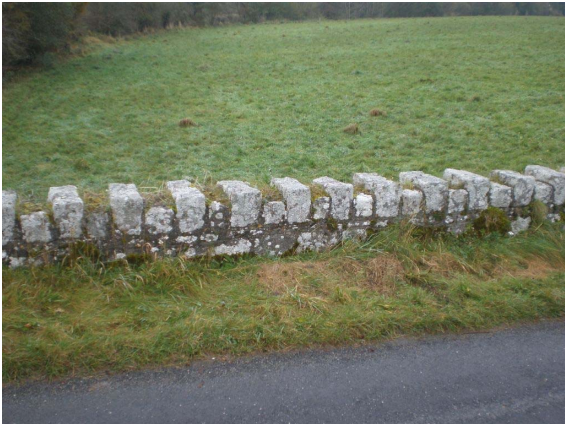
Plate 61 – Cow and calf coping of the abutment wall
