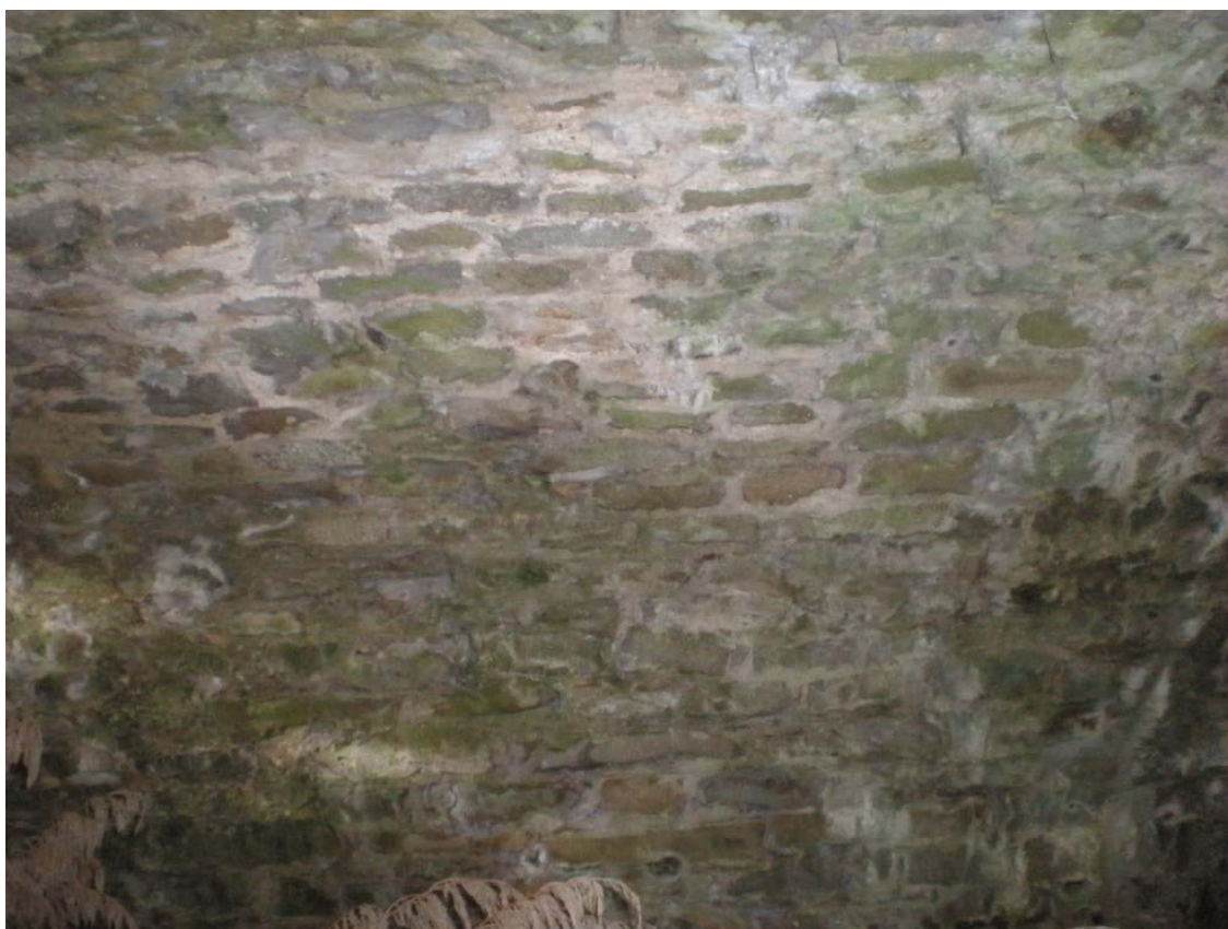
Plate 95 – Dressed granite barrel with lime mortar construction
