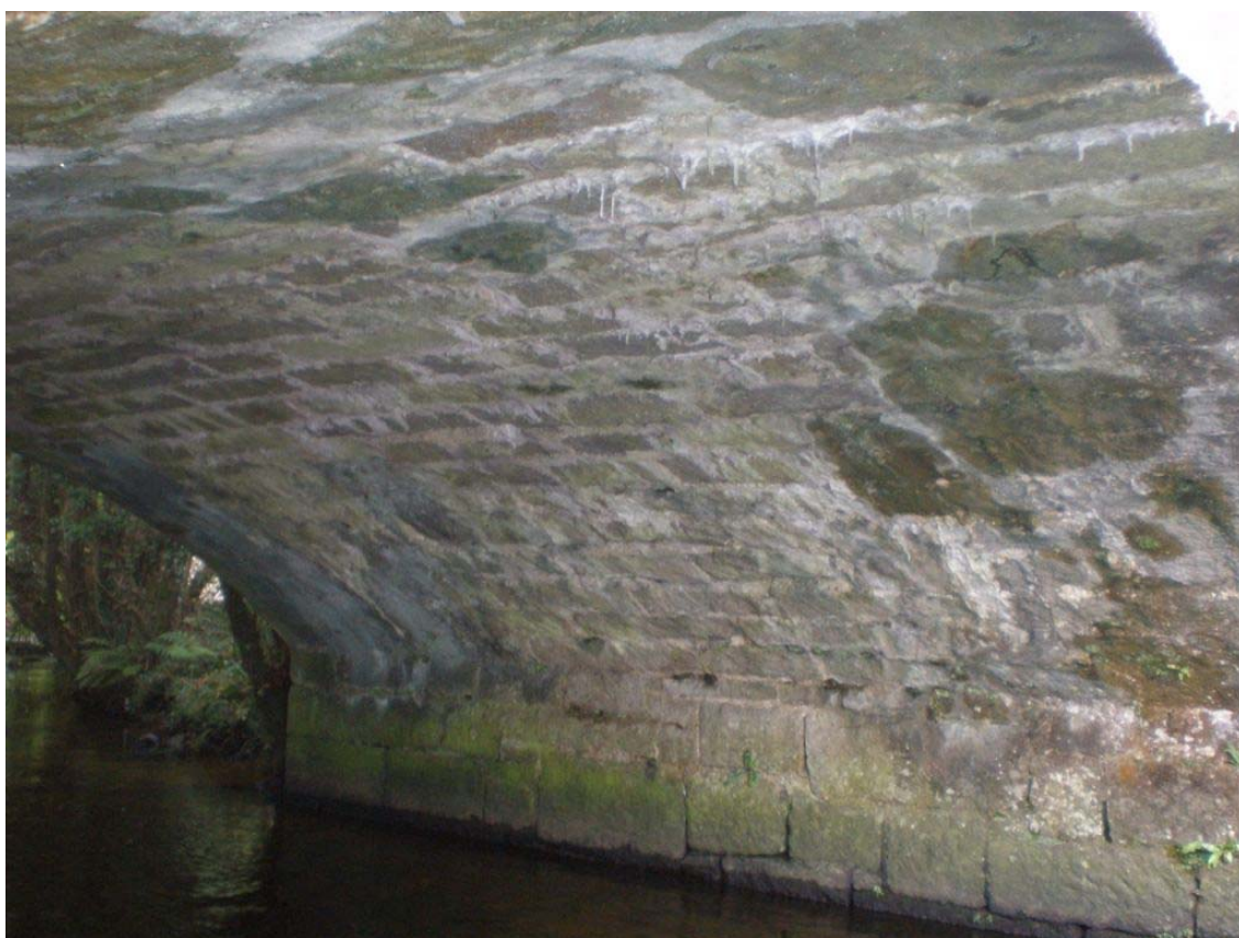
Plate 83 – Impressive, dressed granite barrel, supported by granite abutment
