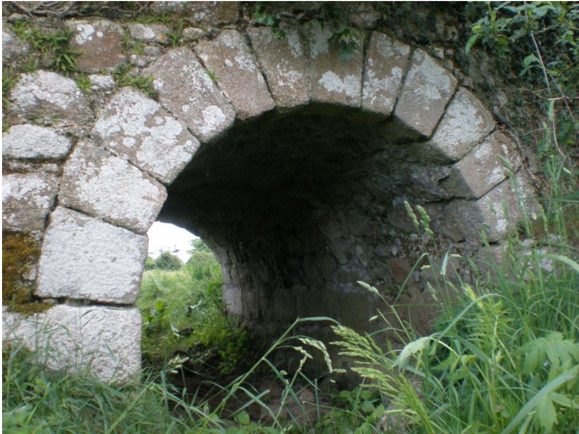
Plate 60 – Dressed voussoirs of side arch
