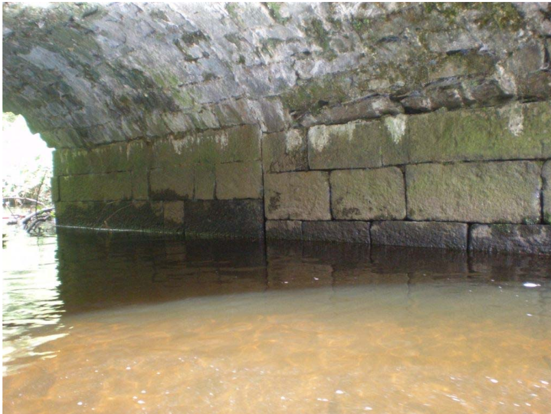
Plate 32 – Distinct line showing different phases of construction at Bunnahown Bridge
