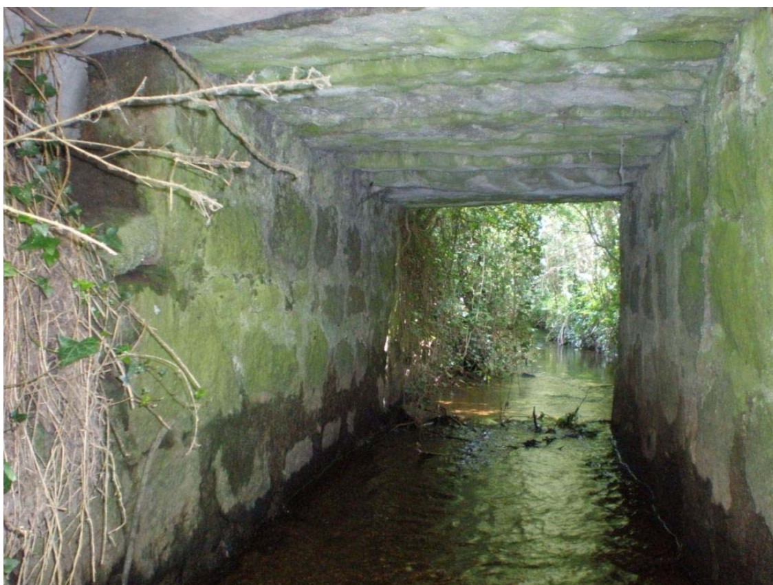
Plate 63 – View from the river bed of one of the arches, note granite lintels
