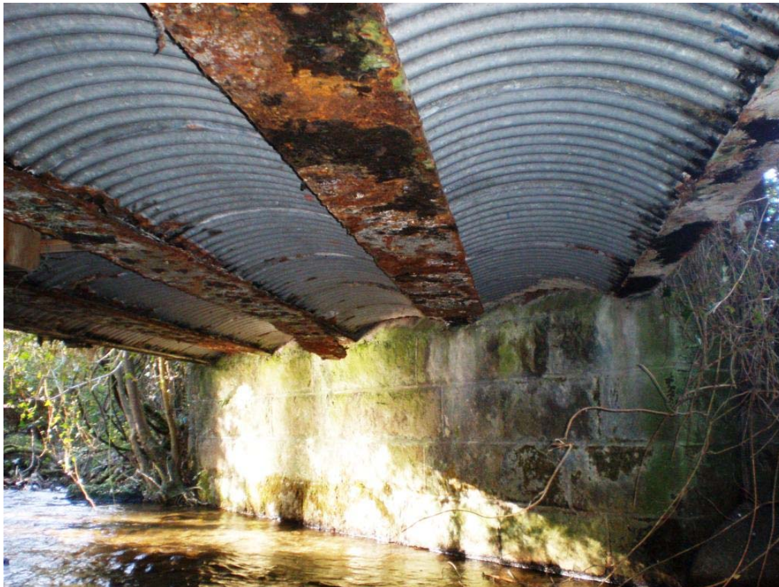
Plate 36 – Ashlar abutment, with steel beams and corrugated iron forming the Jack arch
