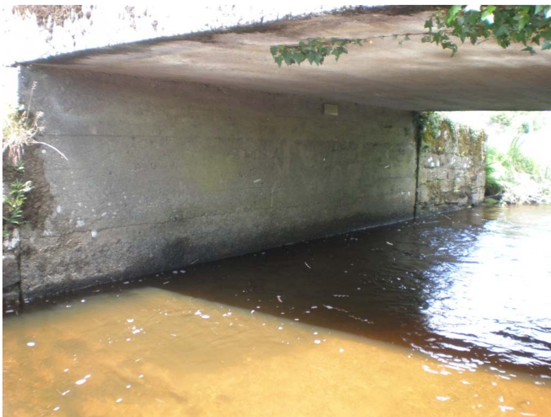
Plate 72 – Outline of timber formwork on abutment and soffit of Knockullard Bridge
