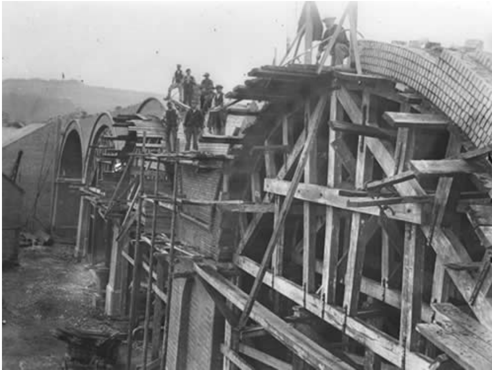
Plate 100 – Example of timber centring in bridge construction
