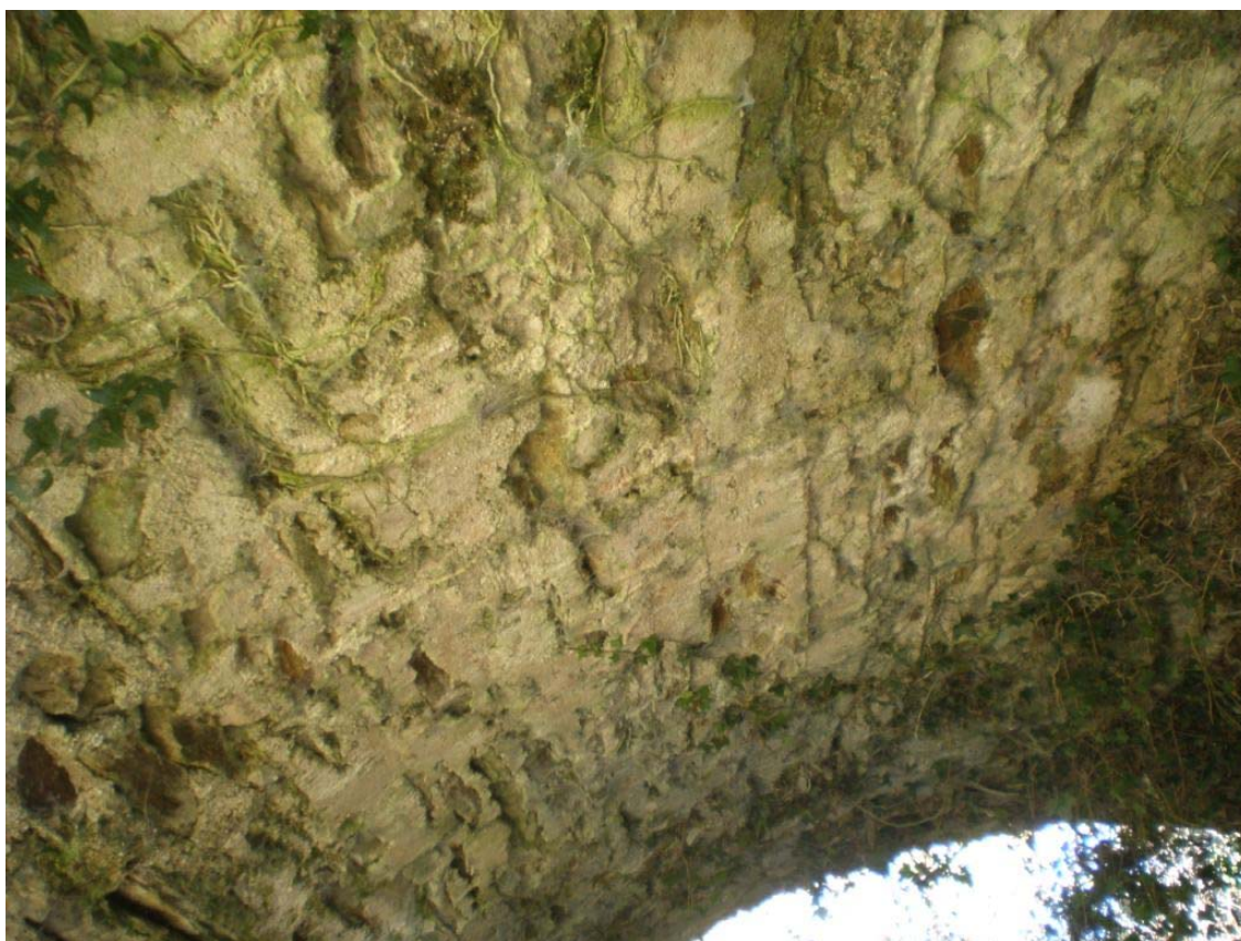
Plate 9 – Outline of centring remains on the barrel of Rosdellig Bridge
