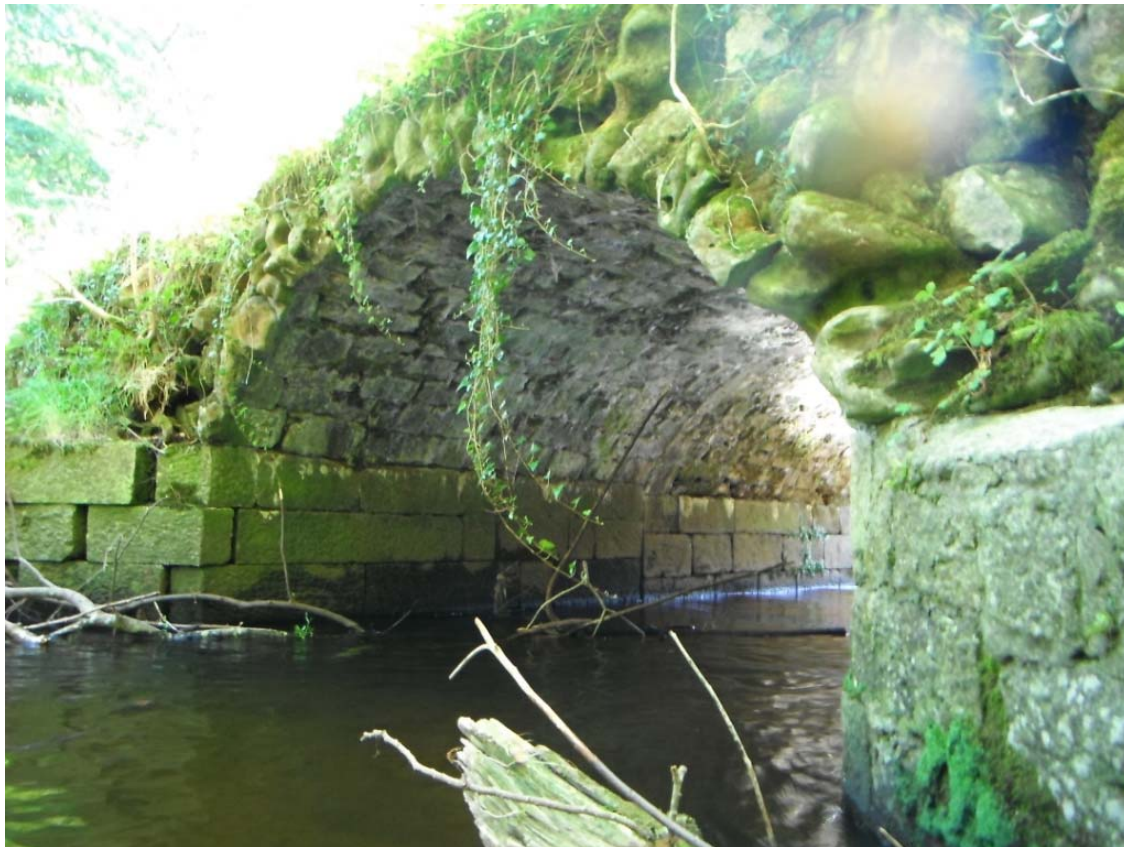
Plate 30 – Central arch with ashlar pier and dressed barrel
