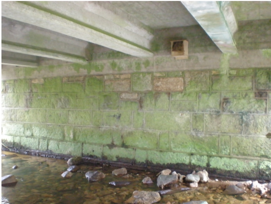
Plate 51 – Finely dressed, granite ashlar abutment, with trabeated steel reinforced beams
