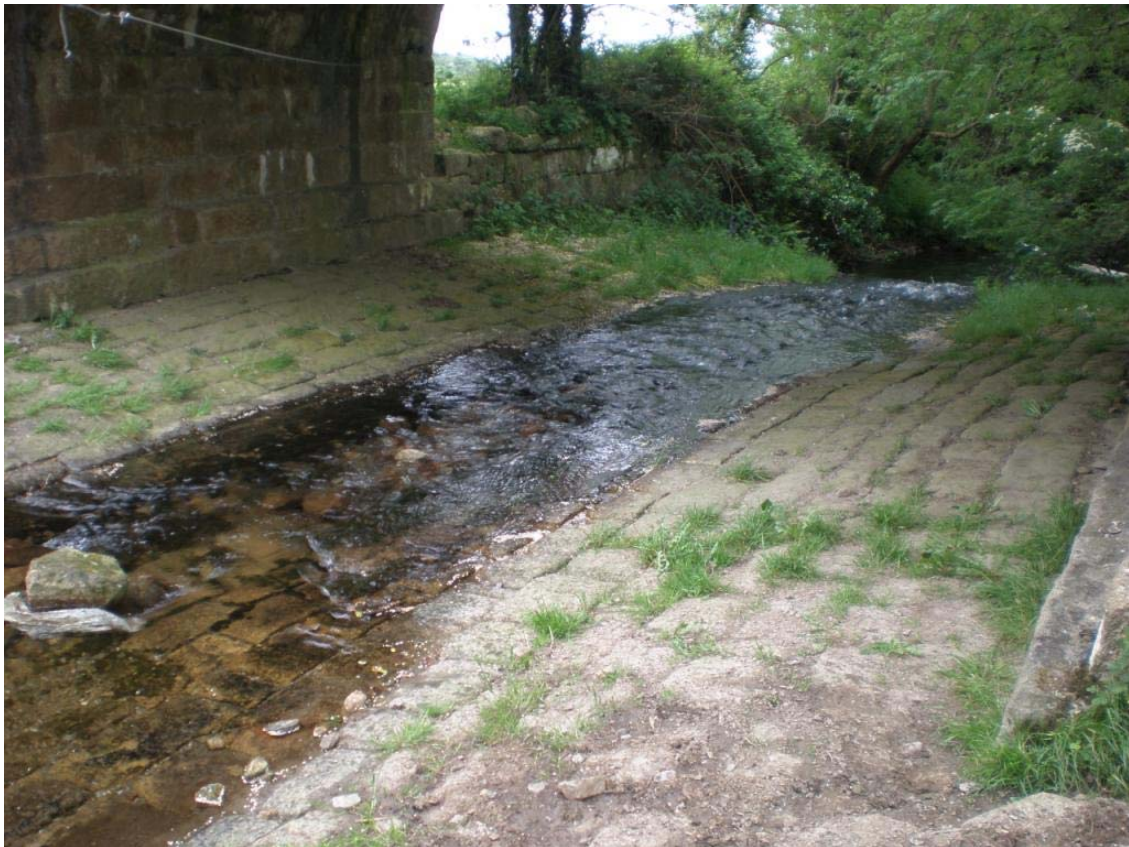
Plate 39 – Concave, granite paved river bed
