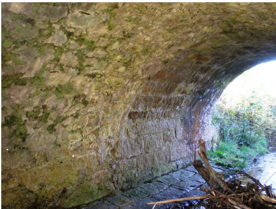
Plate 42 – Contrast of new and old abutment and barrel
