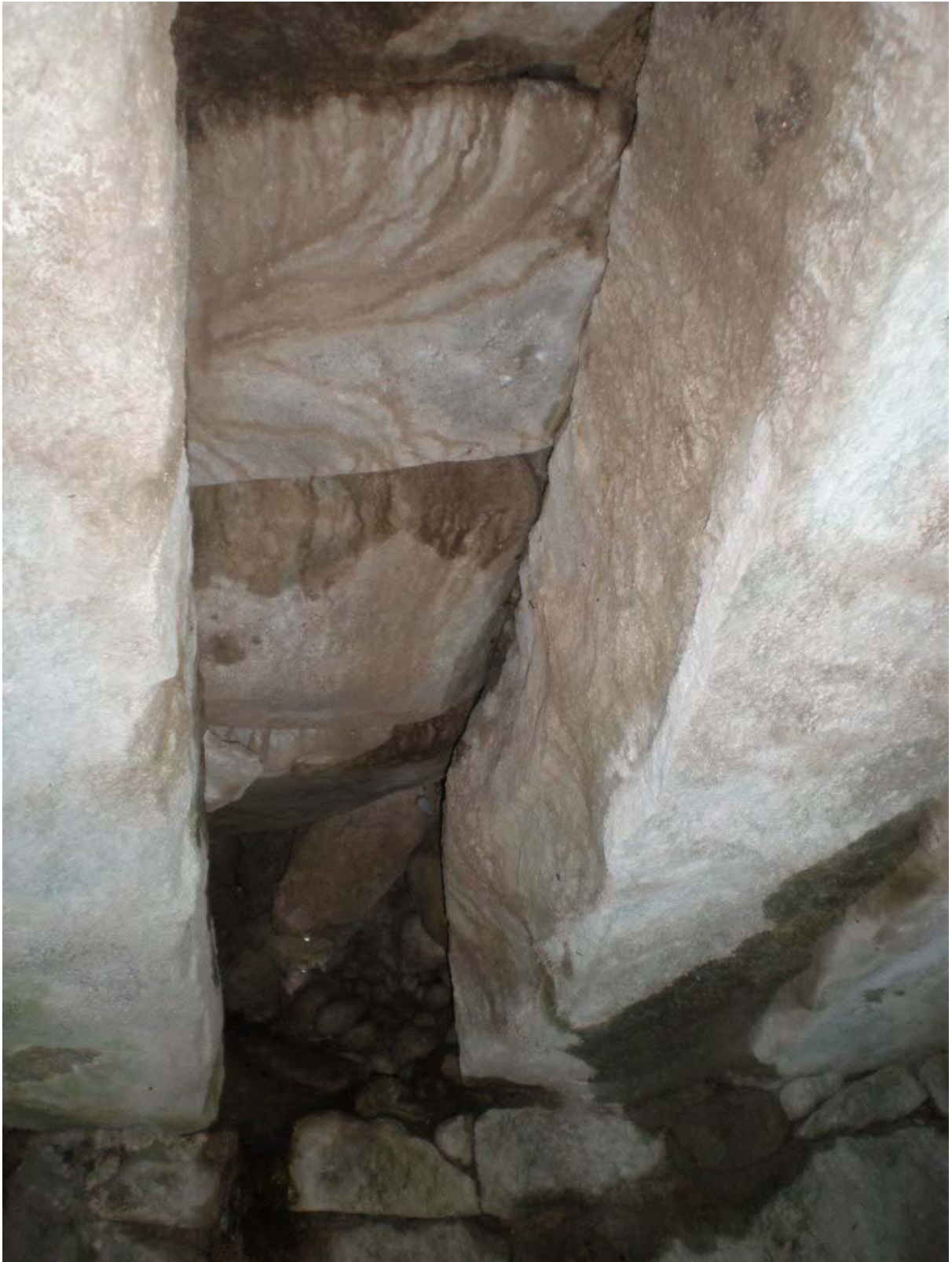
Plate 22 – Missing lintel in soffit, note the lattice style construction
