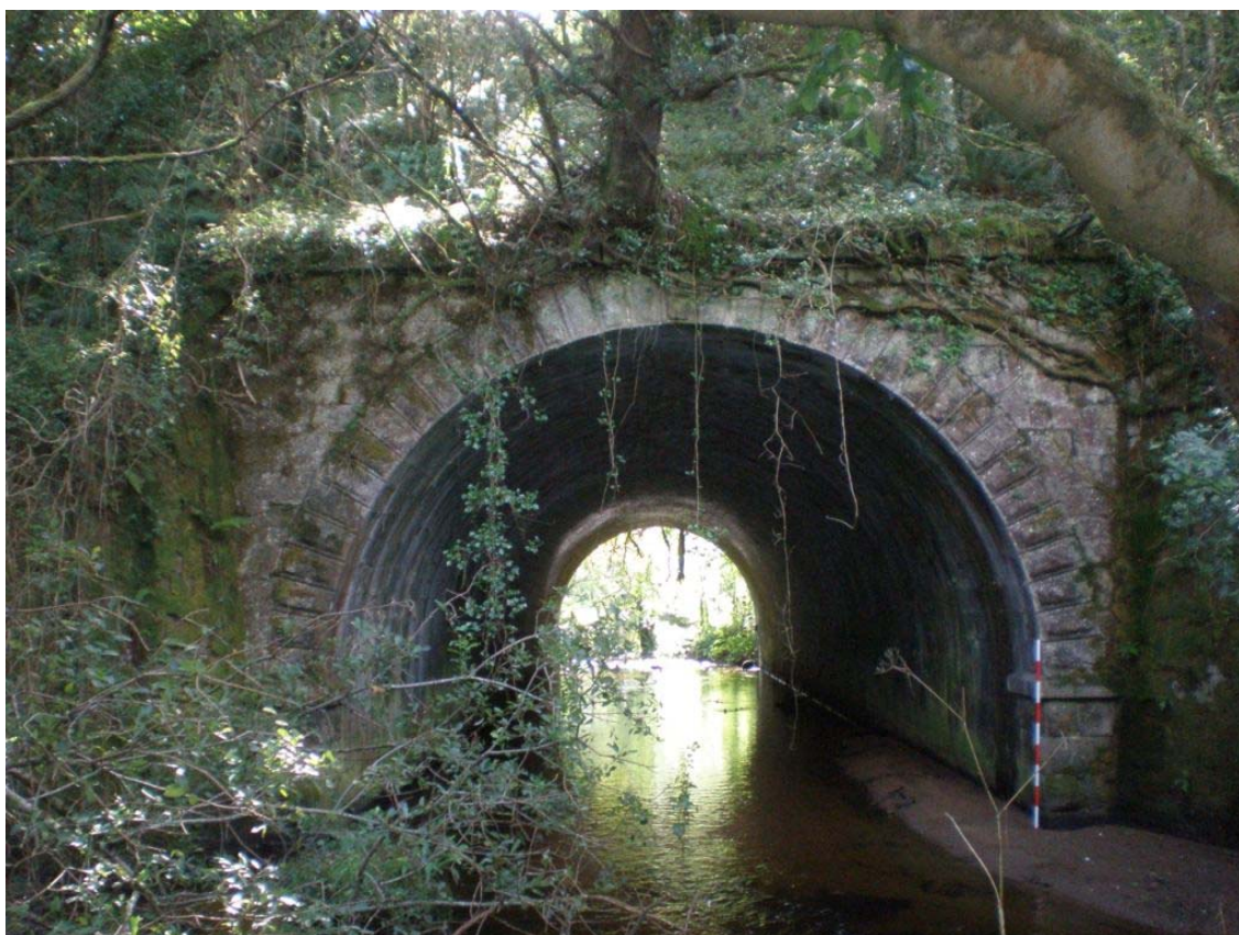
Plate 89 – North-eastern elevation, with all features of finely dressed granite
