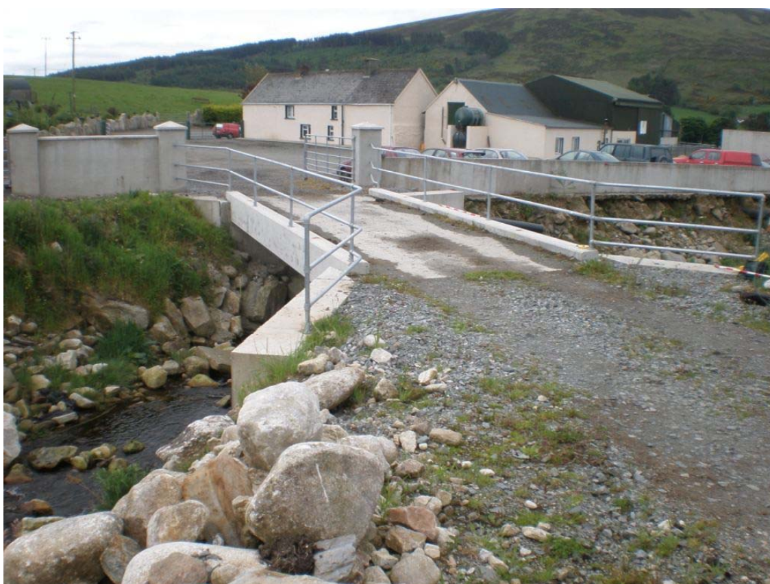
Plate 45 – Surface view of Wards Bridge, note deep scouring of the banks
