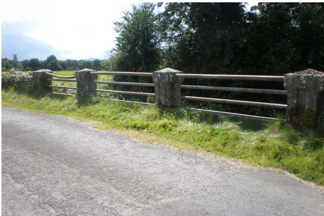
Plate 78 – Concrete post and railing parapet on the road
