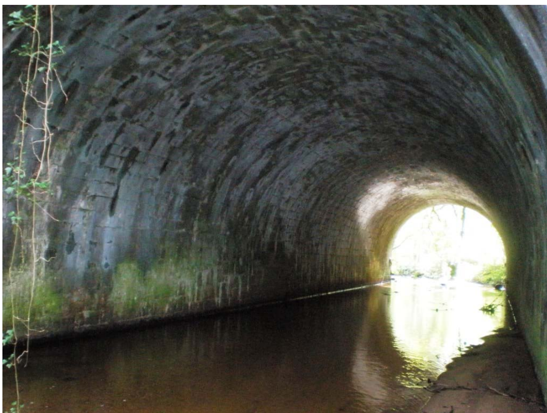
Plate 90 – Finely dressed granite barrel, built to courses
