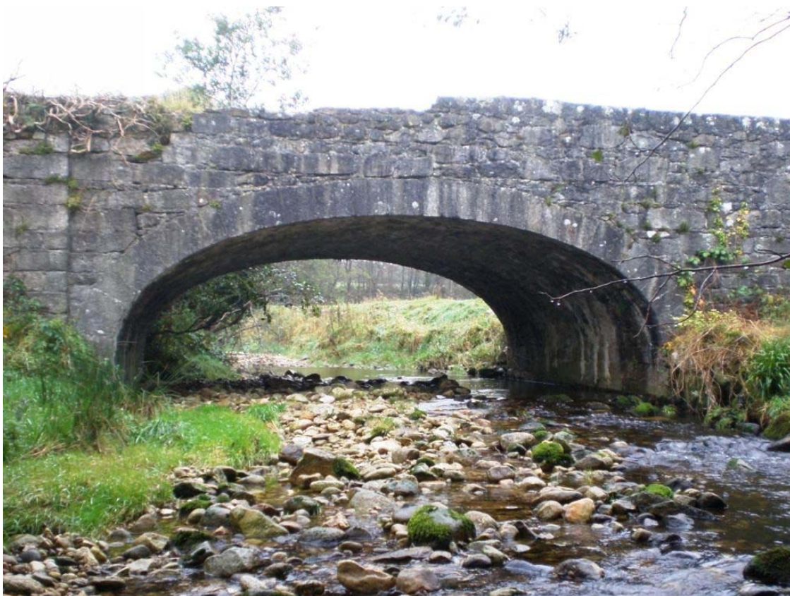
Plate 46 – South elevation of Scullogue Gap Bridge, with missing coping
