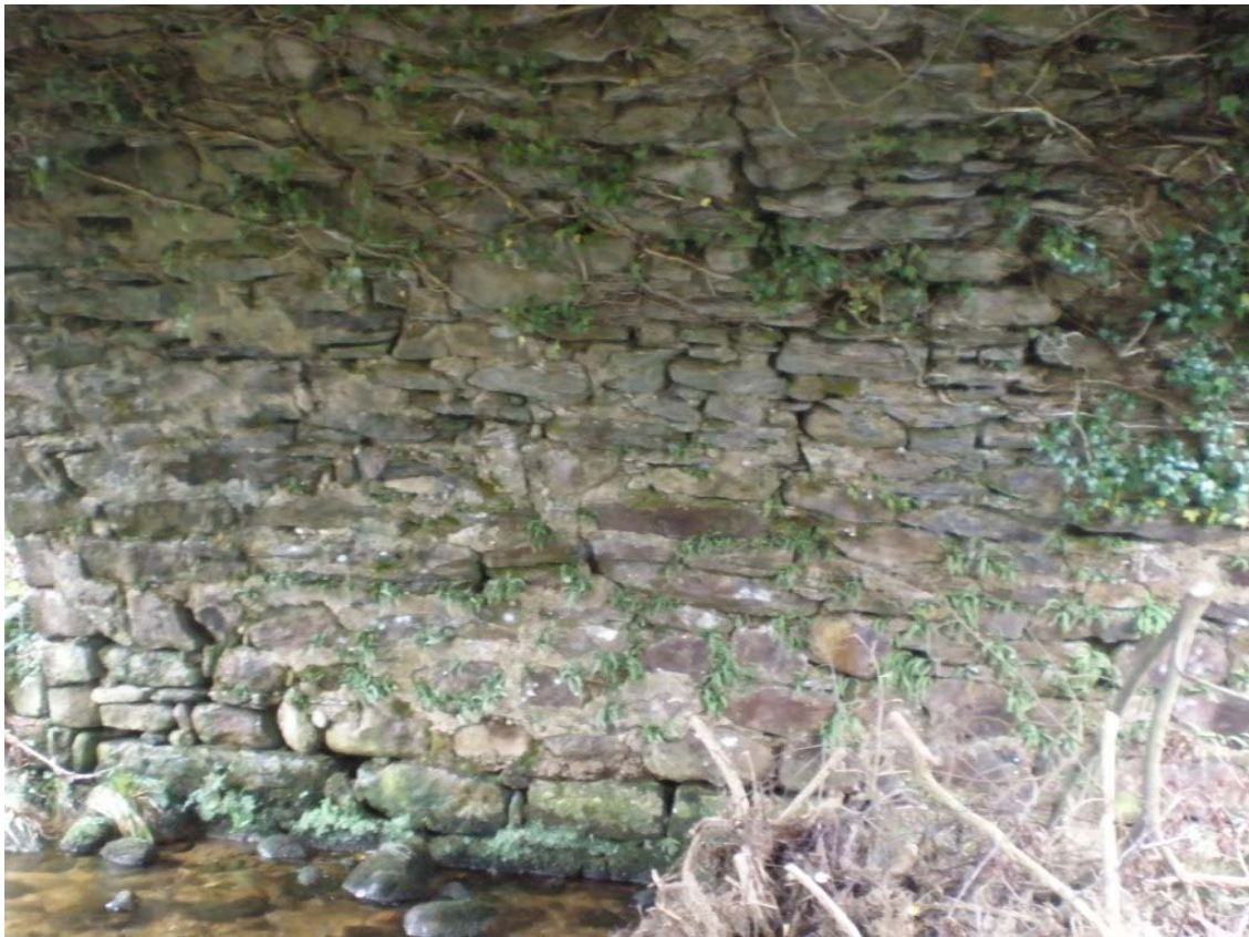
Plate 4 – Random rubble construction of barrel and abutment
