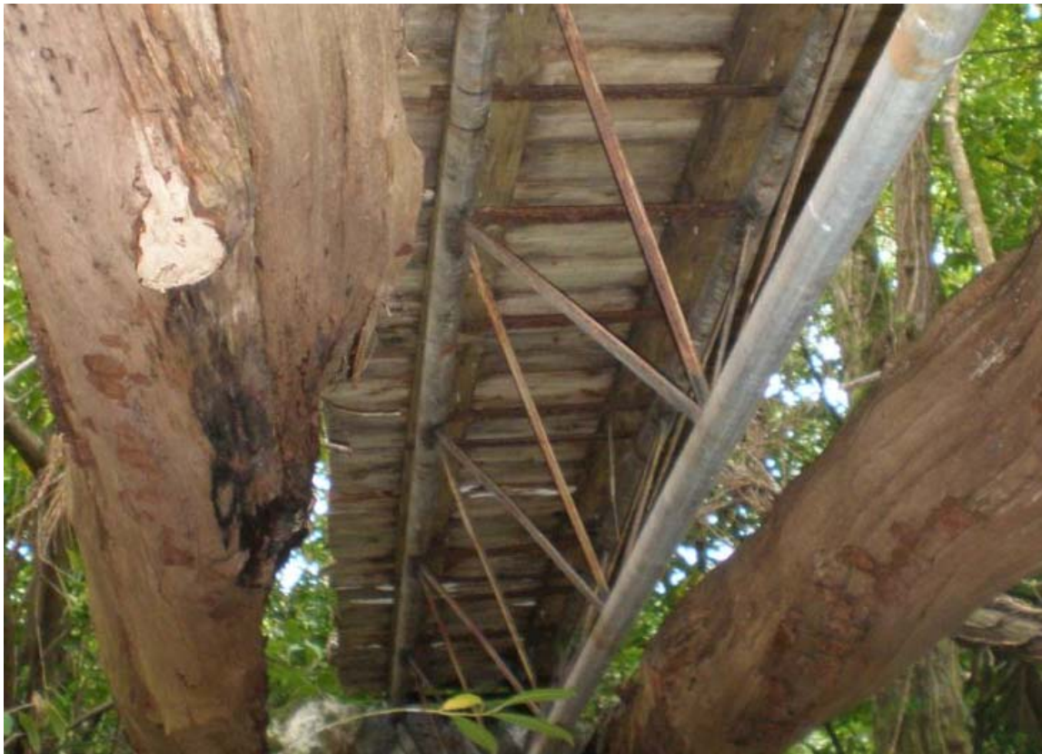
Plate 26 – Tubular framework for Foot Bridge
