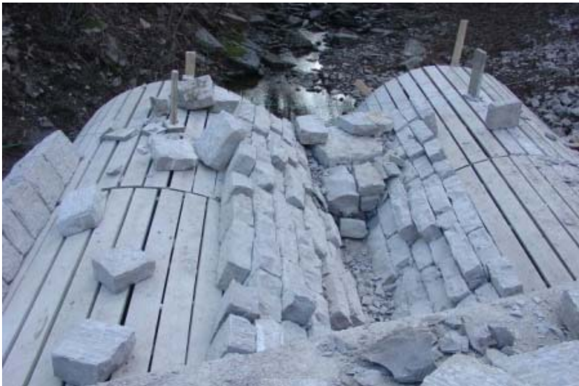
Plate 99 – Timber centring from above courtesy of http://www.drystone.org/
