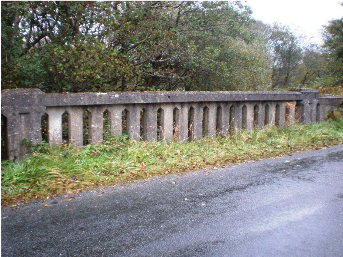
Plate 52 – Concrete balustrade as parapet on the road
