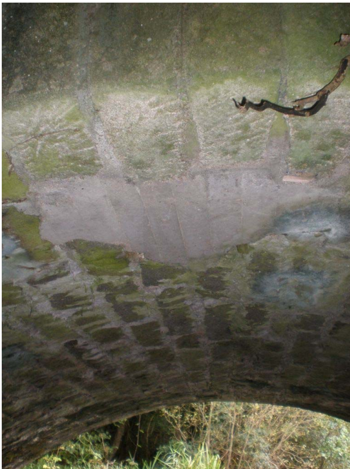
Plate 84 – Barrel of bridge, with later cement remedial work. Is this related to the attempted destruction of the bridge?
