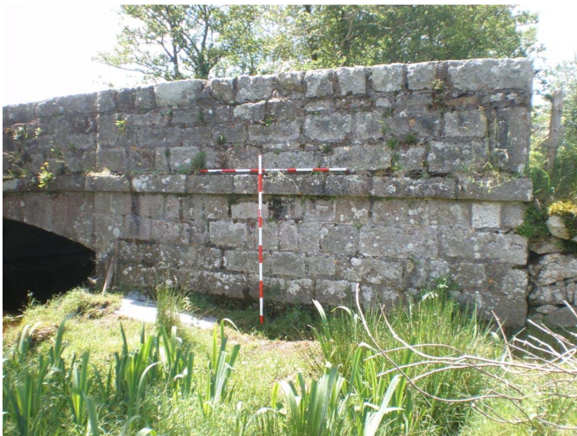
Plate 69 – Eastern elevation of dressed granite abutment and string course
