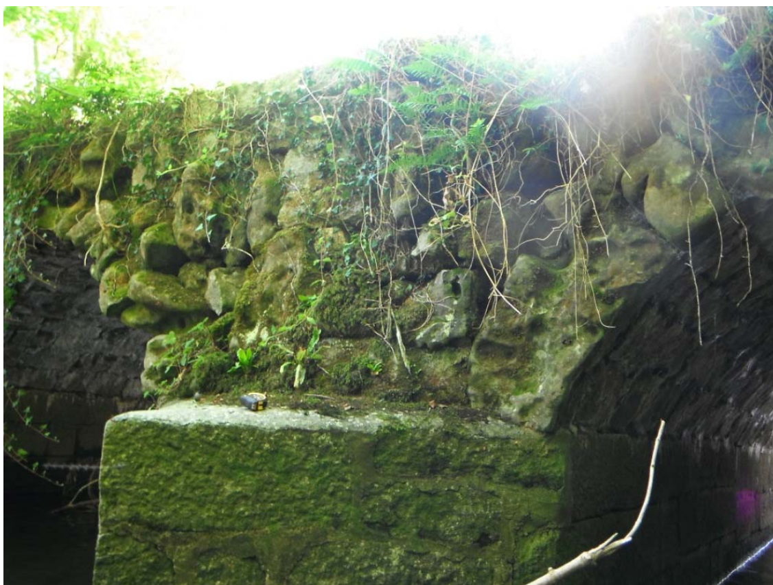
Plate 31 – Random rubble spandrel, with triangular cutwater
